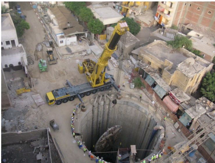
Figure 10: Aerial view with recovery of cutting wheel
