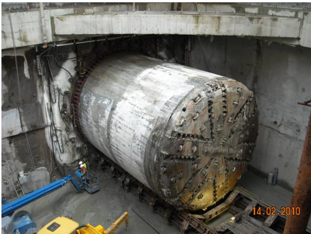
Figure 3: Rescued tunnel boring machine
