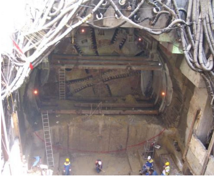
Figure 9: Opened diaphragm wall
