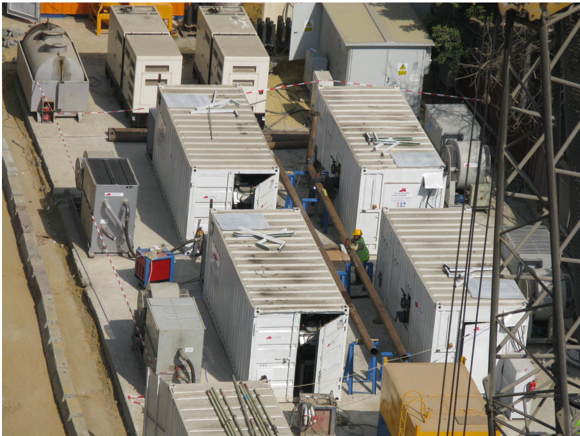
Figure 8: The four freeze plants for the Metro Cairo project
