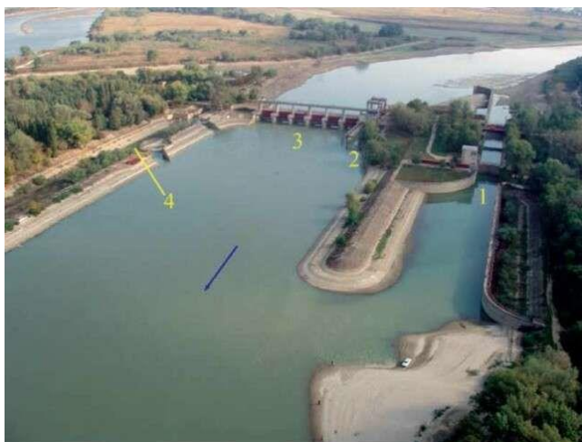
Figure 10: Fedorovskiy dam on the Kuban River. 1 – ship lock; 2 – fish lock; 3 – spillway; 4 – technical passage Soldatov (From Pavlov and Skorobogatov 2014)
