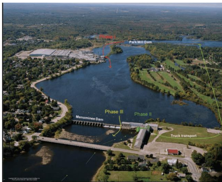
Figure 15: Menominee and Park Mill Dam sturgeon passage facilities (truck transport upstream of the Park Mill dam). Phase I, downstream passage at Park Mill was constructed in 2013-2014 and completed in January 2015; Phase II, an upstream elevator and sorting facility at Menominee was constructed in 2014-2015 and placed in service in 2016; Phase III, the downstream passage at Menominee was constructed in 2016 and began operating in 2017; The upstream pointed arrows denote the upstream migration/movement of lake sturgeon. Photo credit: Eagle Creek Renewable Energy
