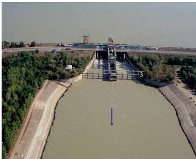
Figure 11: The Krasnodarskiy dam on the Kuban River. 1 – spillway; 2 – mechanical fish lift; 3 – electric barrier for fish (From Pavlov and Skorobogatov 2014)
