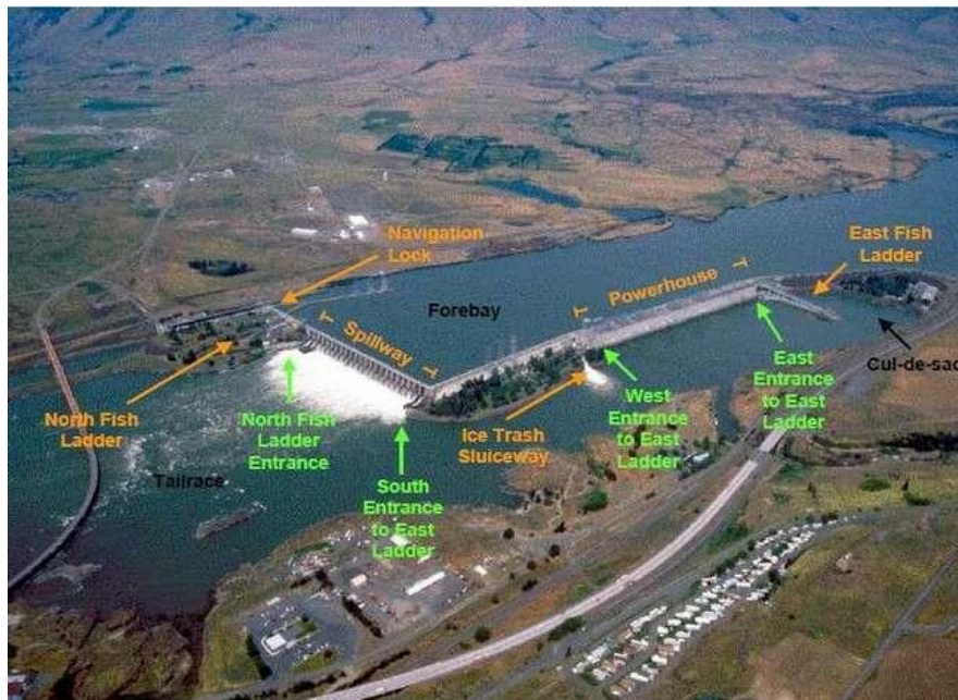
Figure 25 : The Dalles dam with north and east fish ladders (Parsley et al. 2006)
