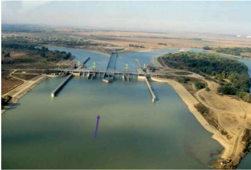
Figure 9: Tikhovskiy dam with fish locks. 1 – ship locks; 2 – fish locks (From Pavlov and Skorobogatov 2014)
