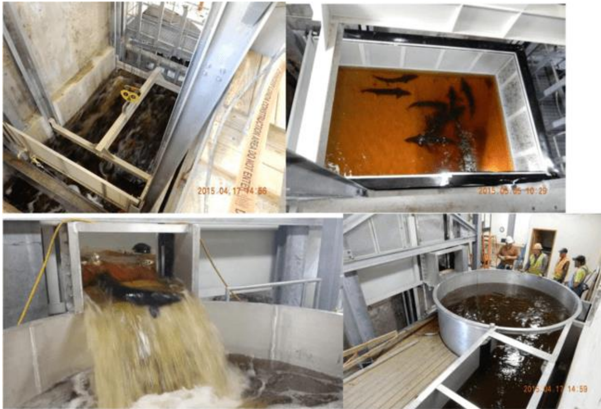
Figure 16: Upstream fish lift and sorting facility. Photo credits: Rob Elliott, U.S. Fish and Wildlife Service
