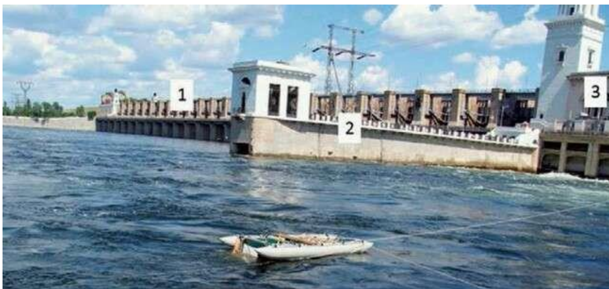
Figure 8: Tsimlyanskiy dam on the Don River. 1 – overflow dam; 2 – fish lift (trapping pool); 3 – powerplant (From Pavlov and Skorobogatov 2014)
