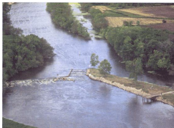
Figure 17: Three-step plunge pool fishway constructed on the Eureka dam in 1988 (From Bruch 2008)
