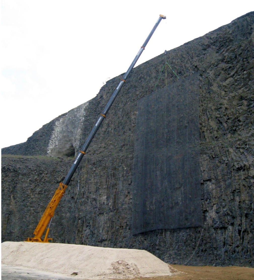
Figure 3. Rock Wall in the South of the Landfill
