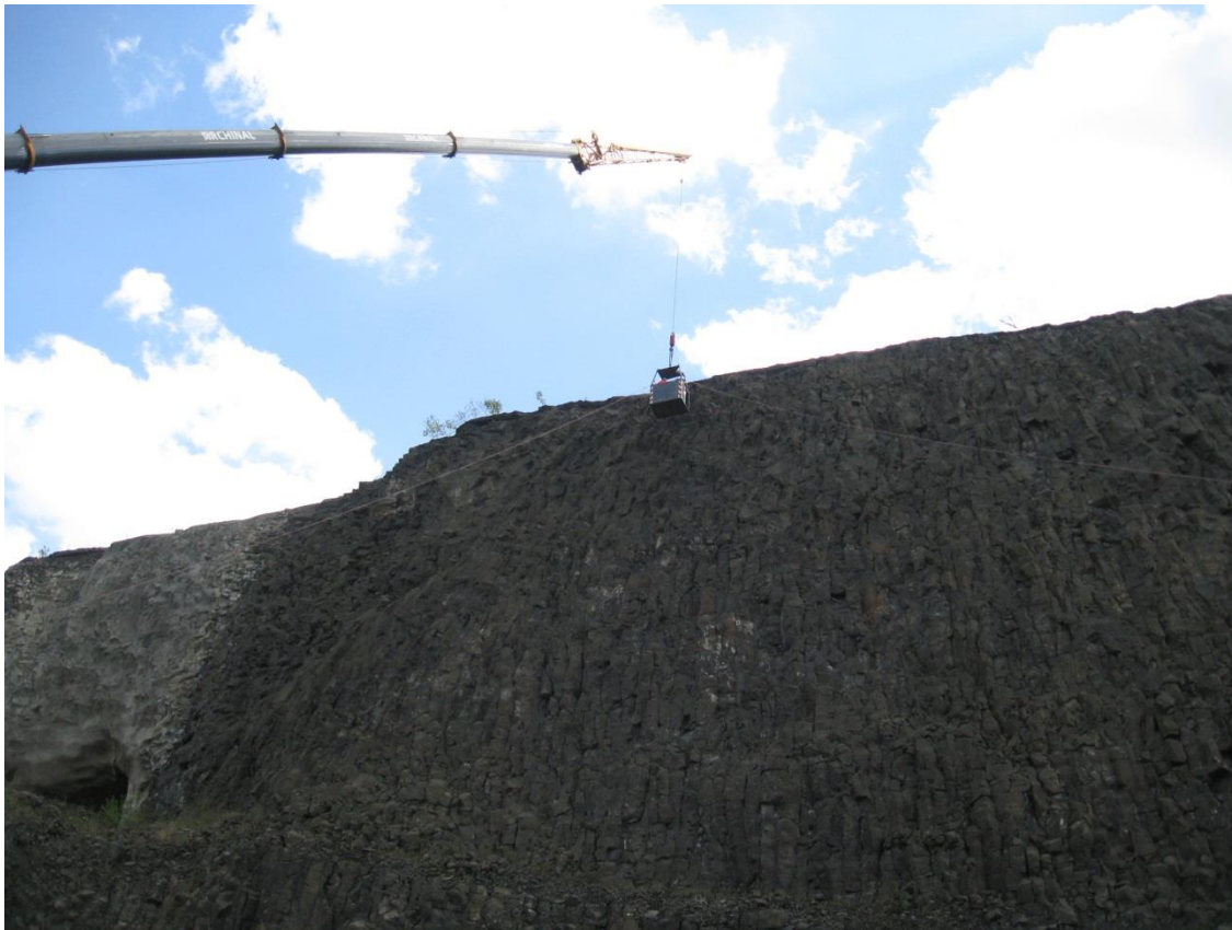
Figure 6. Inspections Along the Rock Wall
