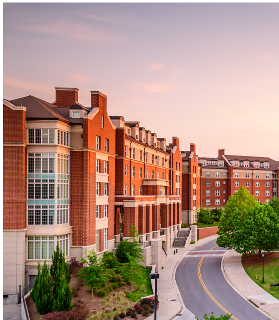
Managers of facility campuses
